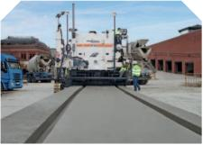
The concrete slab produced by the SP 500 and 3D technology precisely meets the specified requirements
