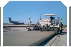
Surface finish using a finishing beam and super smoother
