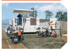
Concrete spreading by means of a spreading auger in a country road project
