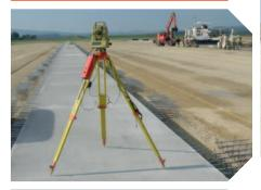
▲ The total station uses sensors to track the prisms mounted on the SP 500, thus calculating the 3D position of the mould
