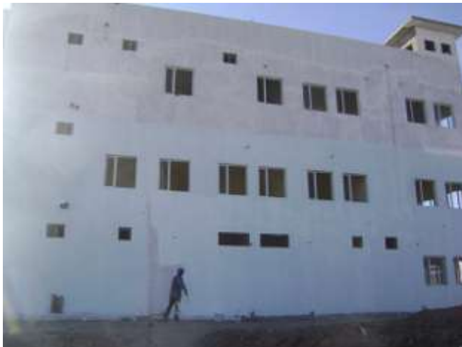
Building Exterior Painting
