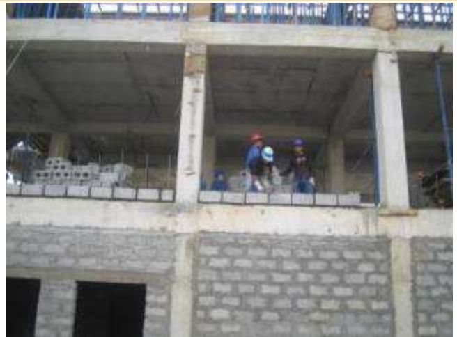
Masonry Work For the Second Floor
