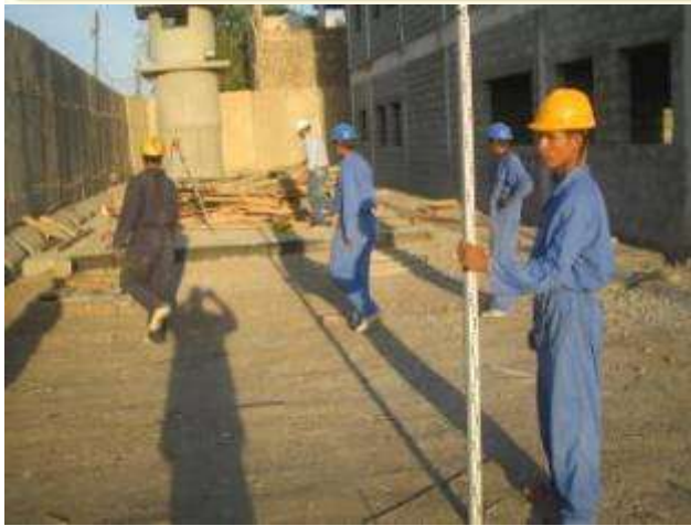
Preparation For Concrete Park Around The Building
