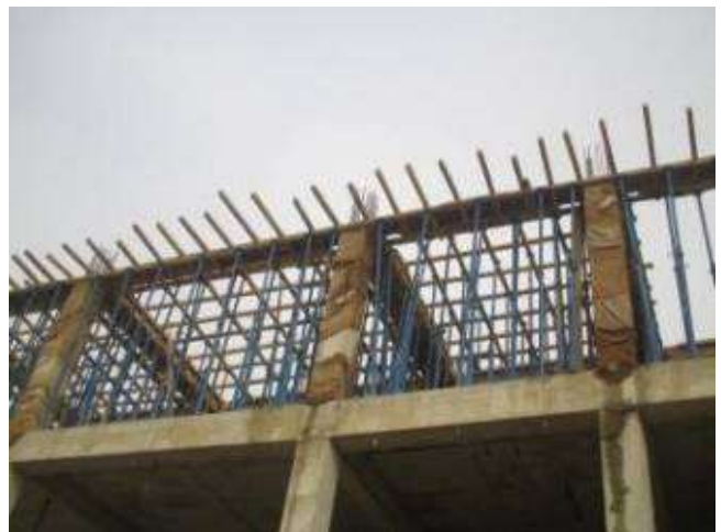
Forming For 3 rd Floor Roof
