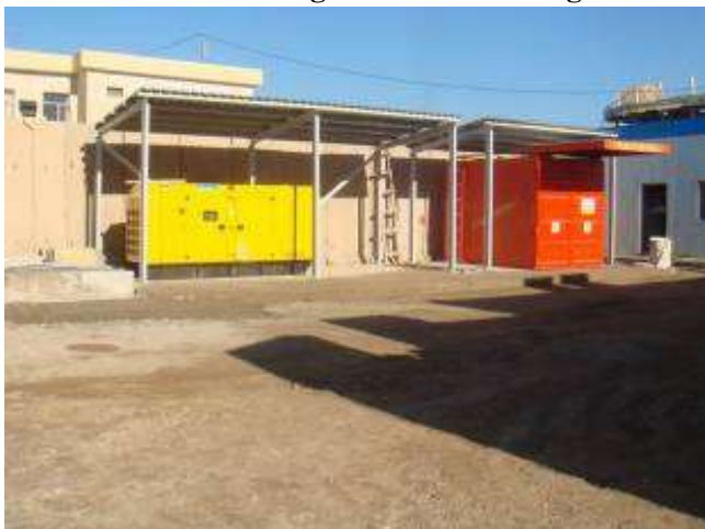
Back Up Power Station And Fuel Station
