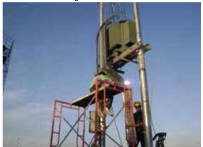
Installing Transformer For The LPS 3
