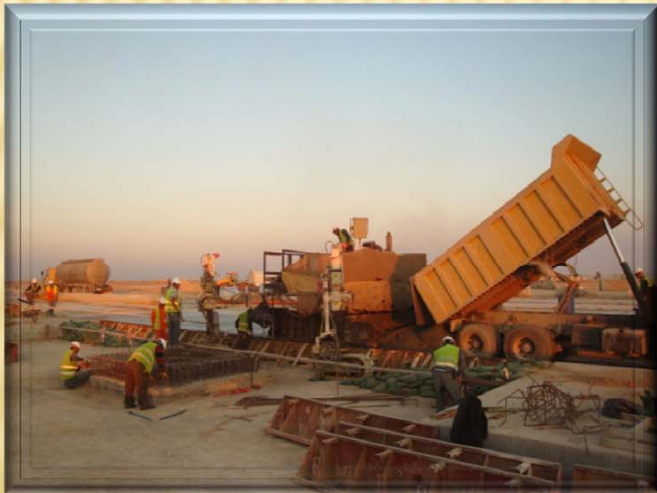
Damping concrete
